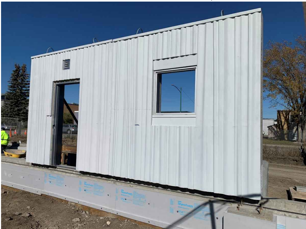
10/10/2023 – Exterior Precast Mockup
