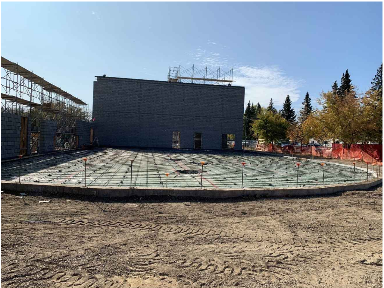
9/29/2023 – Gym Floor Rebar & South Wall
