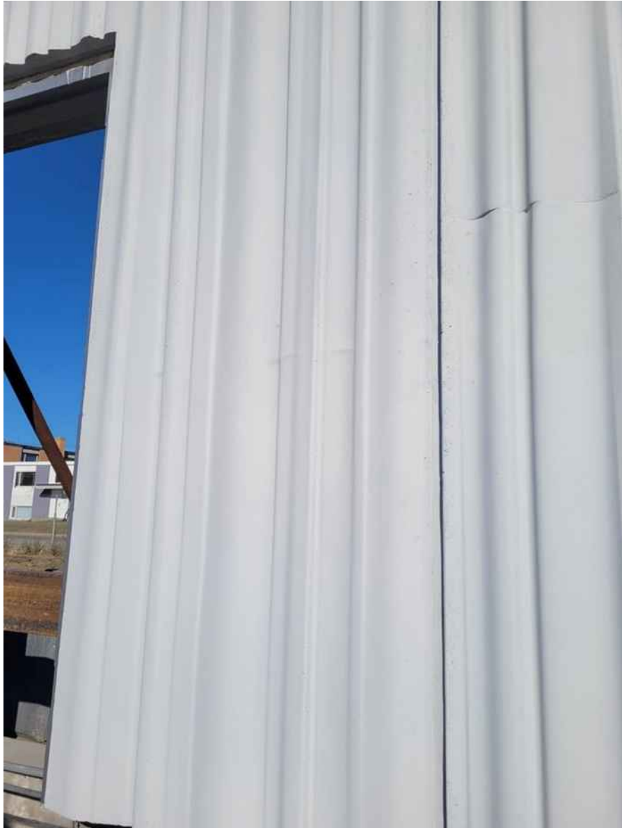
10/10/2023 – Exterior Precast Mockup Staining Closeup
