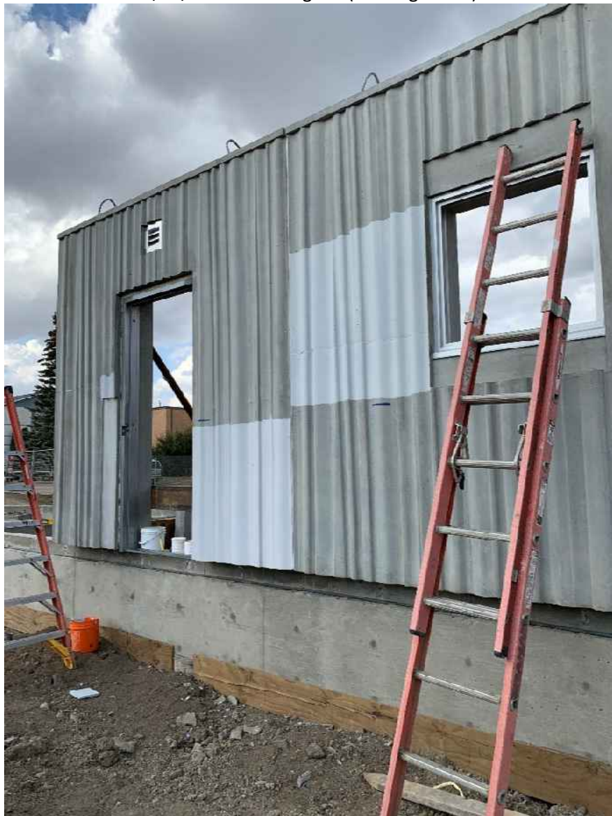
9/29/2023 – Precast Exterior Wall Mockup
